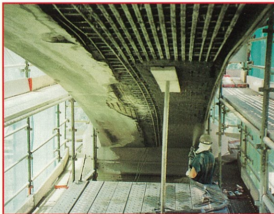
▲ Spraying SikaCrete-Gunite-103 onto the arches.
